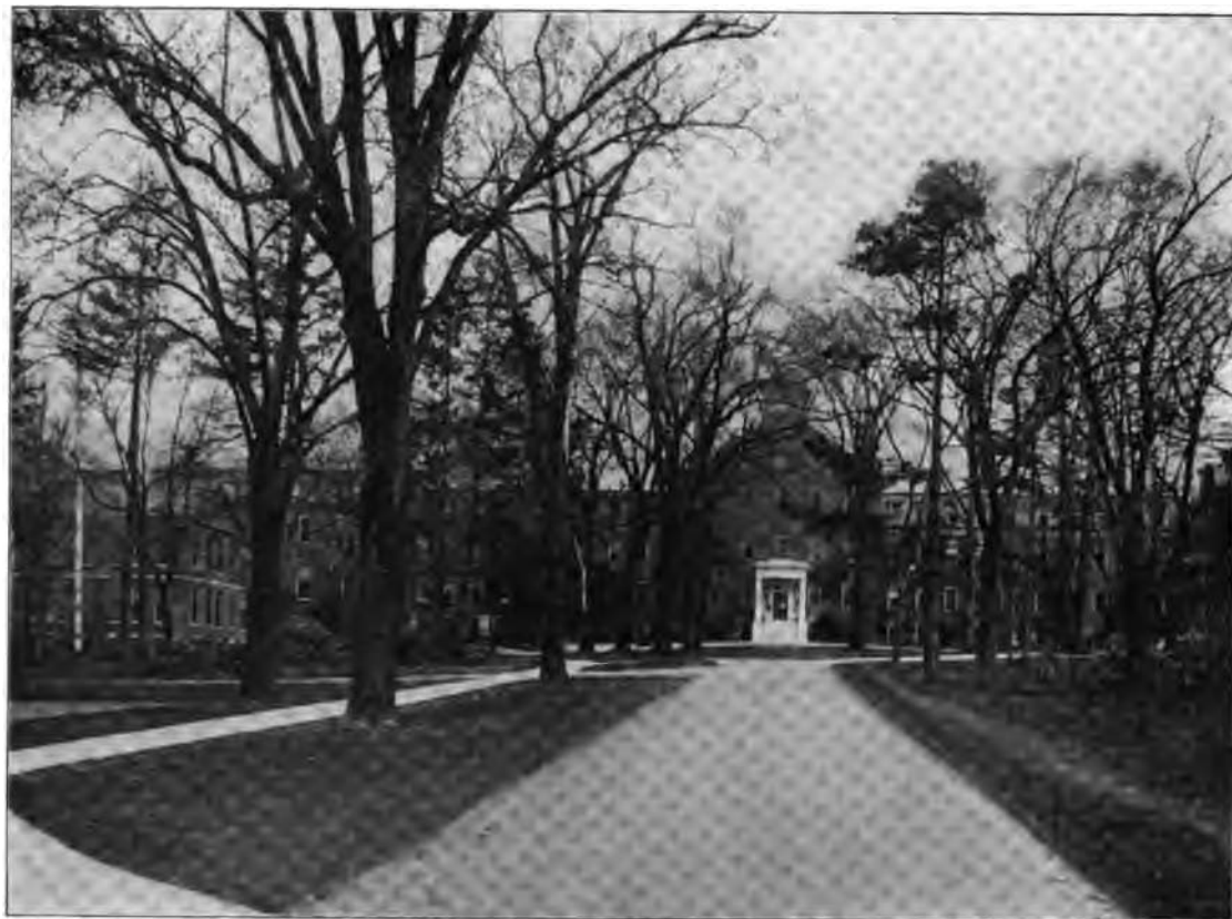
PRESENT FRONT VIEW LOWER SCHOOL BUILDING ON LEFT
