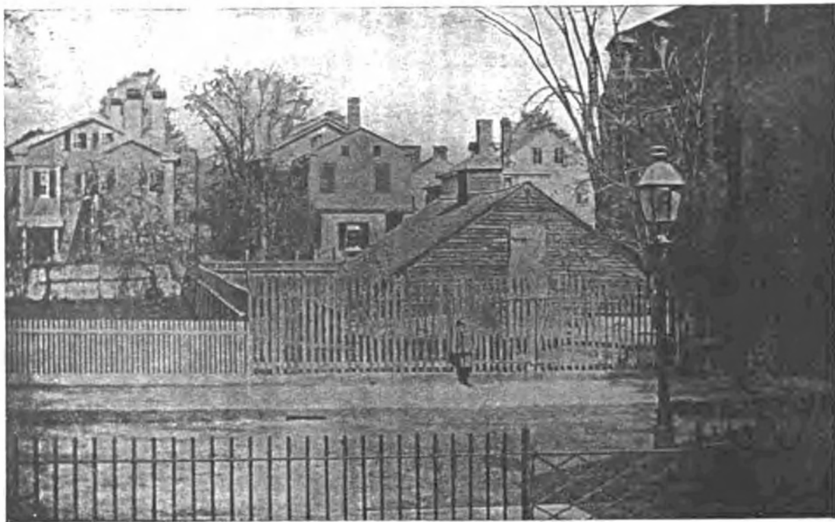
FIELD FOUNTAIN, CLIFFORD STREET, PROVIDENCE. ESTABLISHED IN 1772 FOR THE PURPOSE OF SUPPLYING A PORTION OF THE TOWN WITH WATER. BUILDING DEMOLISHED IN 1900.
