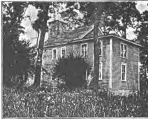
COREY HOUSE, ERECTED 1718, QUIDNISSET, NORTH KINGSTOWN.
