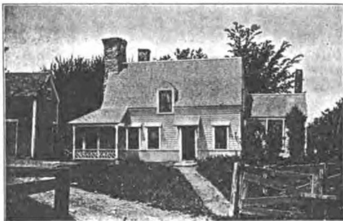
EDWARD MANTON HOUSE, MANTON, JOHNSTON—ERECTED 1688.
