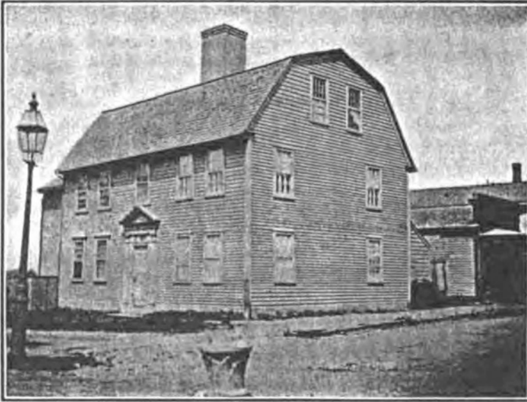
BAKER HOUSE, CORNER WATER AND BAKER STREETS, WARREN.
