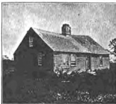
SAUNDERS HOUSE, NEAR ASHAWAY, Erected about 1740.
