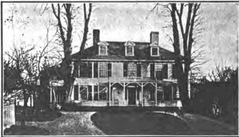
JAHLEEL BRENTON HOUSE, NEWPORT. ERECTED IN 1720.
