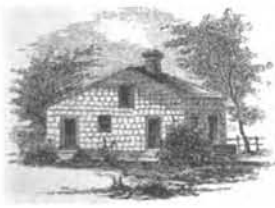
HOOPER'S RESIDENCE AT WILMINGTON
