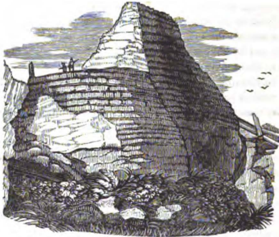
Shift or "fault" in the round tower of Terranuova in Calabria, occasioned by the earthquake of 1783.
