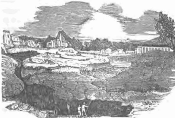
Deep fissure near Polistena, caused by the earthquake of 1783.
