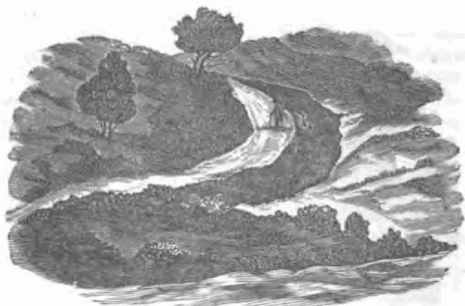
Chasm in the hill of St. Angelo, near Soriano, in Calabria, caused by the earthquake of 1783.
